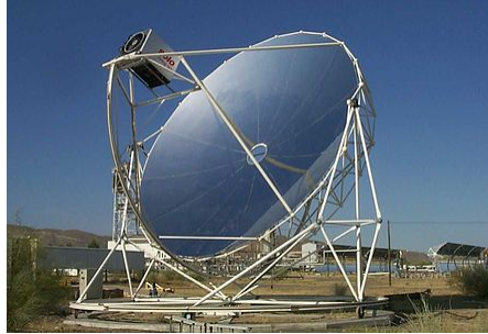
Point focus parabolic mirror with Stirling engine at its centre and its solar tracker at Plataforma Solar de Almería (PSA) in Spain
